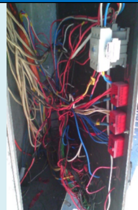
Untidy wiring of Main Switchboard
