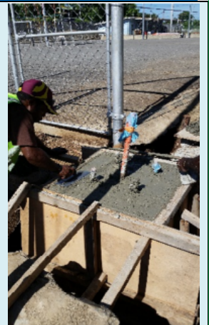
Finishing works on concrete base
