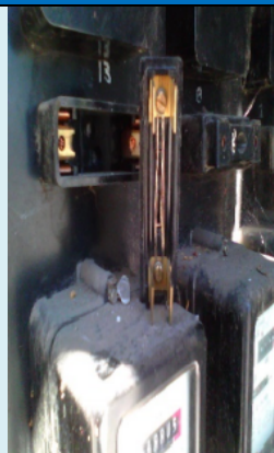
Using copper wire as HRC Fuse
