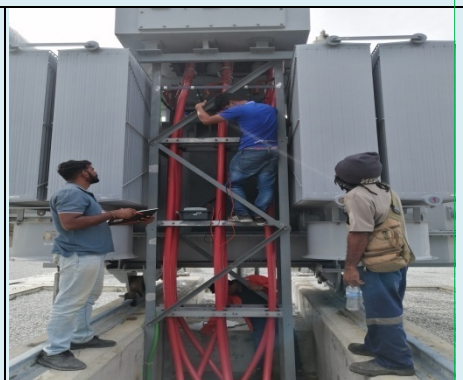
Test engineers confirming correct phases
