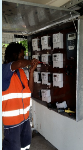
Easypay meter installation
