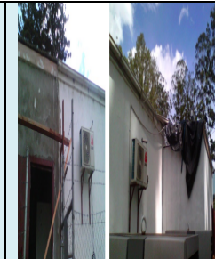
Installed new Split Air-Conditioning systems
