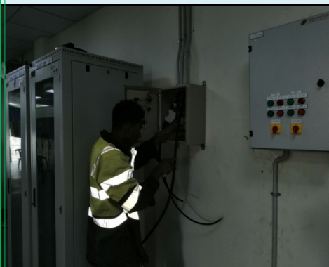
Wiring of power and control boards for A/C split units
