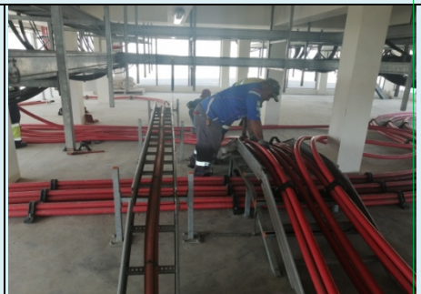
Laying 11kV cables on cable ladders
