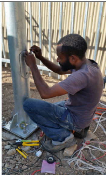
Connecting power supply for CCTV camera & Security flood lights
