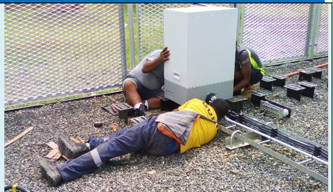
Installation of Communication cabinet
