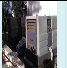
Installation of 90kVA Generator with ATS system
