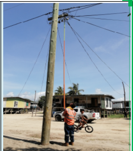
Inserting HRC Pole Fuses
