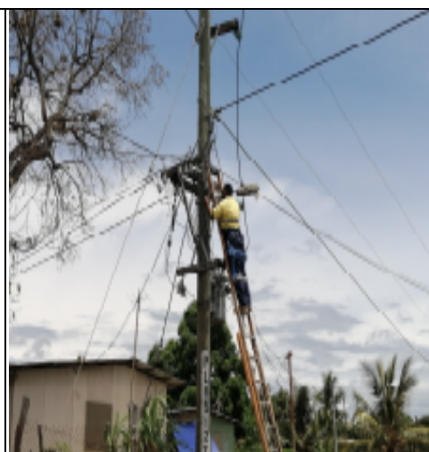
STRINGING OF ABC CABLE TO MAIN PNG POWER POLES
