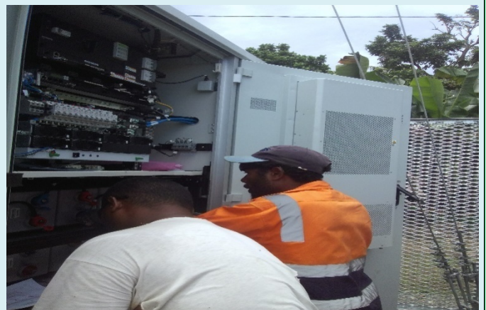
Wiring of Power Cube and Battery Banks
