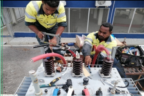
Cable preparations of 11kV transformer
