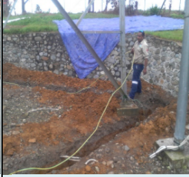
Laying Earthing Grid on tower footings
