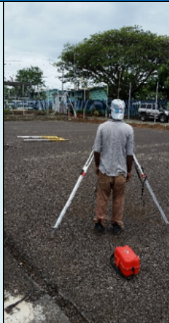
Using dumpy level for courtyard lightings foundations
