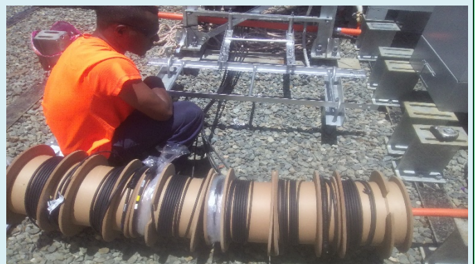
Cabling works for Radio Receiving Units
