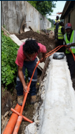
Insertion of DB supply cables into conduit
