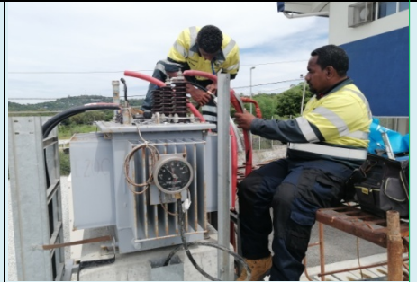
Terminating 95mm 2 HV cable for 11kV transformer
