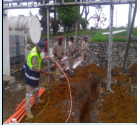
Earthing the building structure
