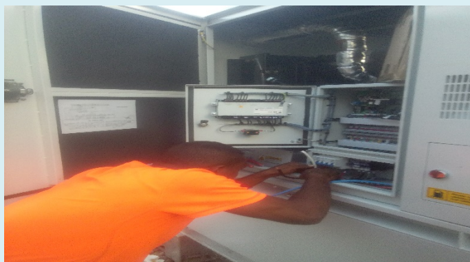
Wiring of Genset Controls
