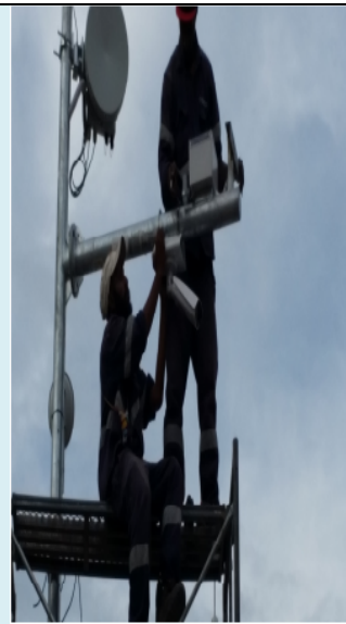
Installing CCTV camera and flood lights
