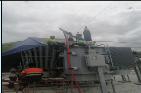
Terminating Neutral conductor on 66/11kV transformer
