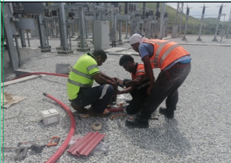
Cable preparations of transformer main Neutral
