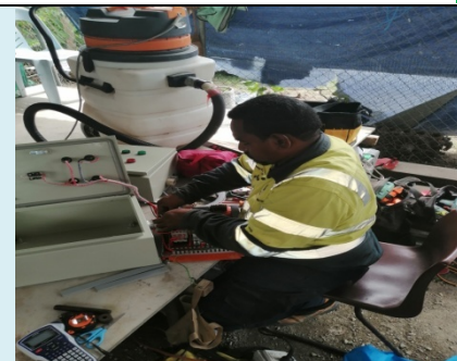
Wiring of A/C Control boards
