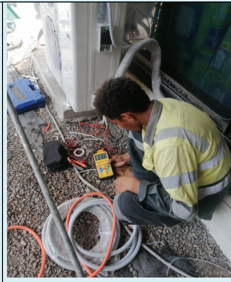
Conducting Insulation Test for the A/C units power supply cables
