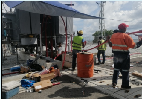
Termination of 630mm 2 HV cable for 66/11 TX-1
