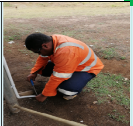
Installing main earth
