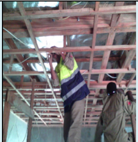
Internal wiring of lighting and power
