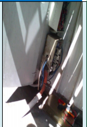
Unsafe & Unprotected live conductors
