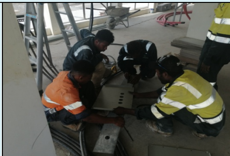
Making cable entry for sub distribution boards
