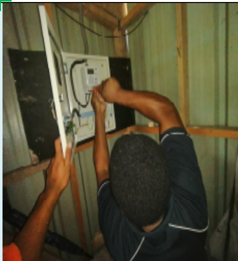
Test & Commissioning MSK units
