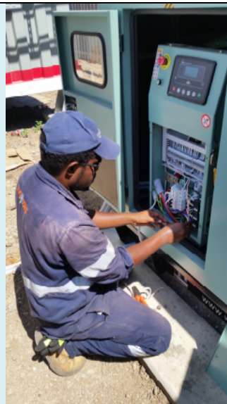
Wiring of 90kVA Genset
