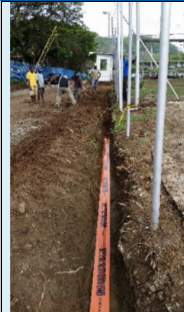
Laying electrical tape for underground conduits
