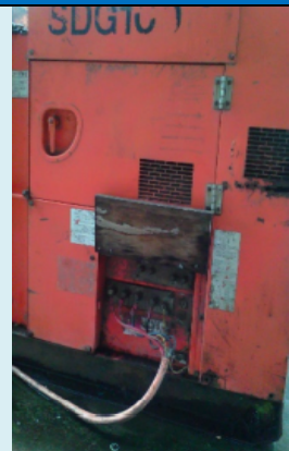
Unsafe bare live wires from genset mains
