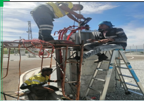
11kV HV cable termination preparations
