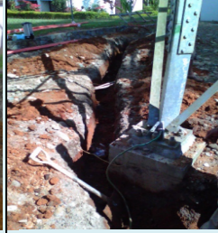
Earthing of tower footings
