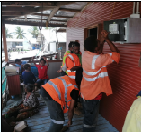
Installing easypay meters
