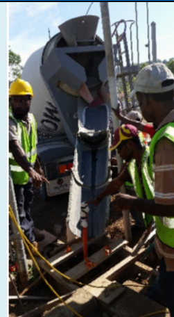
Pouring concrete onto foundation base for court yard lightings
