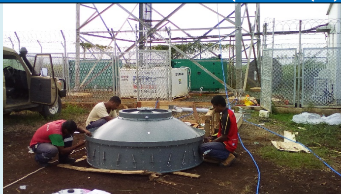
Assembling the Main Link microwave
