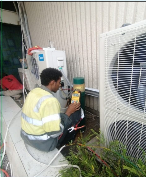
Conducting Insulation Test for the A/C units power supply cables
