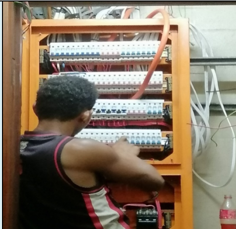
Installing new circuit breakers
