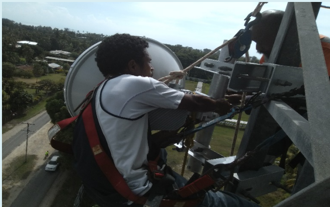
Installation of Microwave antennas
