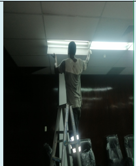
Replacing faulty lights
