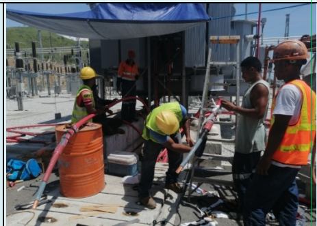
Cable preparations for 630mm 2 HV cable for 66/11 TX-2
