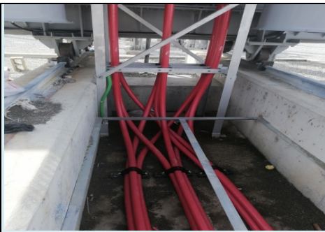
Terminated 11kV HV cables
