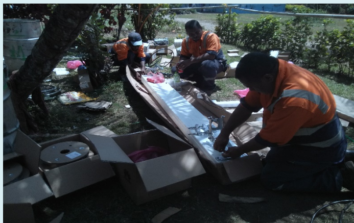
Assembling of Sector Antennas
