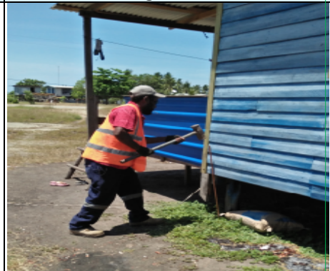
Installing main earth
